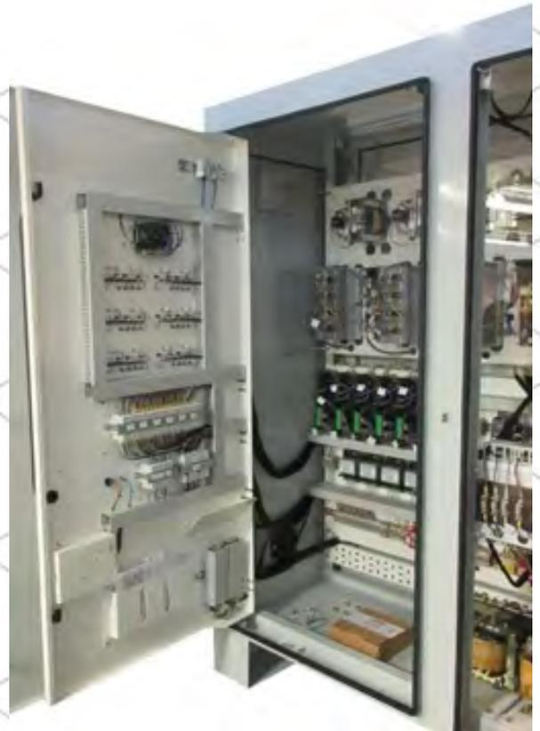
Multi Channel Transformer Rectifier Units
