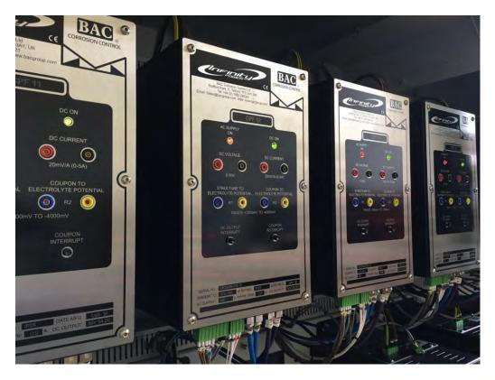
The transformer rectifier is housed inside a cabinet with the control and indication mounted on an internal hinged door. The control box is fitted with a viewing window to enable easy viewing of the control and indication of the rectifier. The user is protected from high voltages via door interlocked isolator
