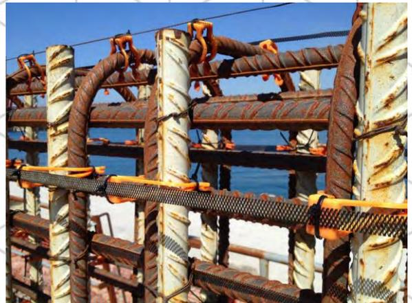
Example of an MMO Ribbon Mesh installation.
