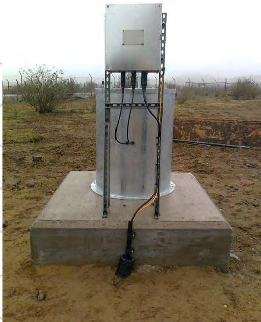
Typical Deep Well Anode Groundbed Installation
