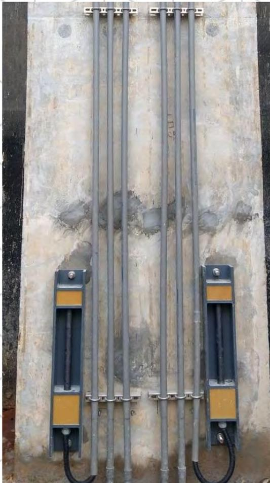
Mixed Metal Oxide Anodes for Water Intake Channel Structures
