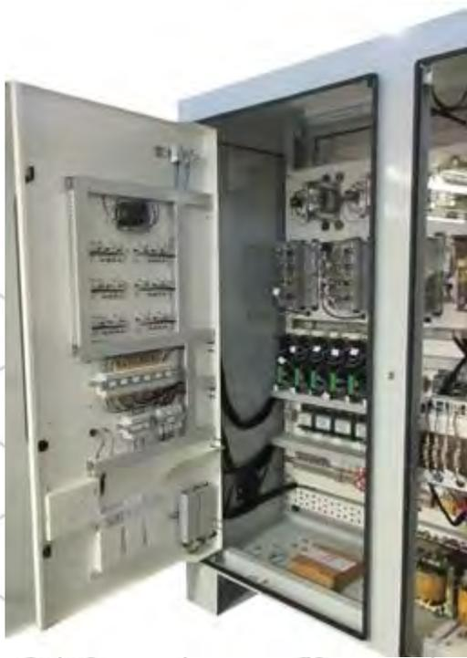
Multi Output Transformer Rectifiers for control over complex plant structures
