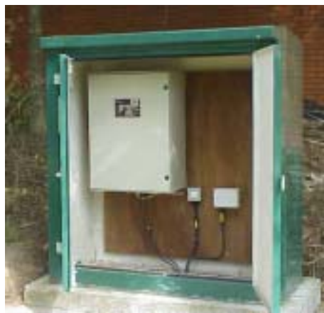
Transformer rectifier installation
