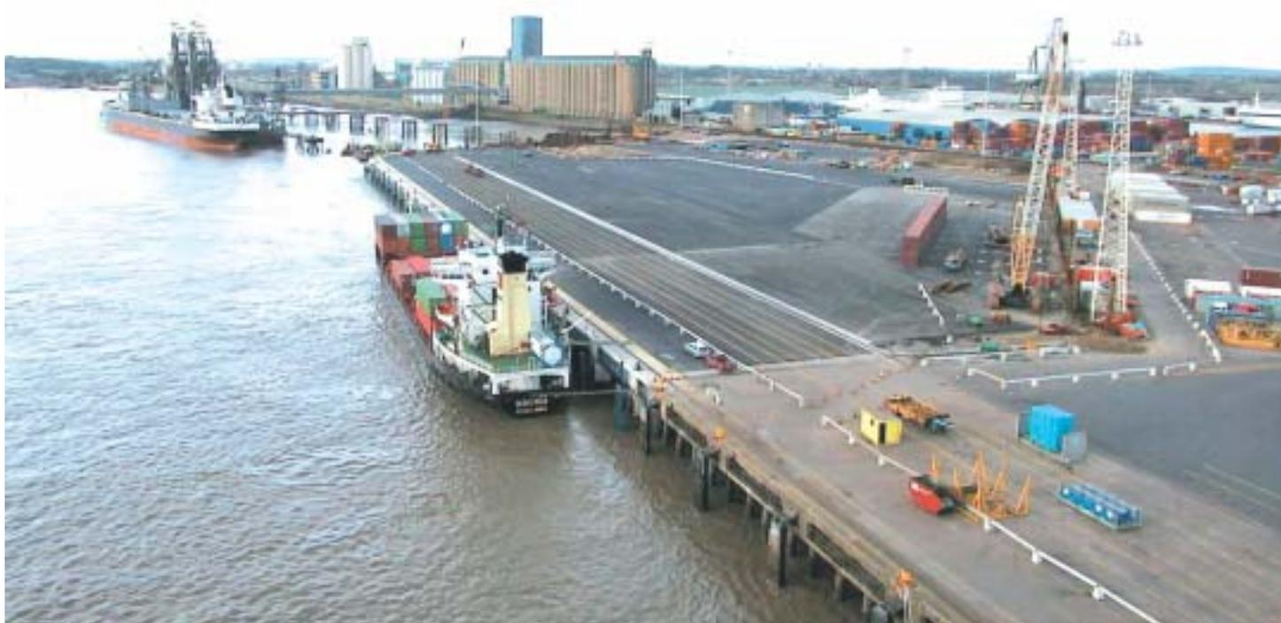
A new 300 metre long deep water Quay under construction at London's Tilbury Docks, for Tilbury Container Services, is to have its steel piles protected against advanced low water corrosion (ALWC) by a BAC Corrosion Control impressed current cathodic protection (ICCP) system.
