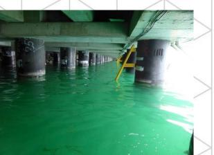
Cantilever Anode Supports for Tubular Pile CP system
