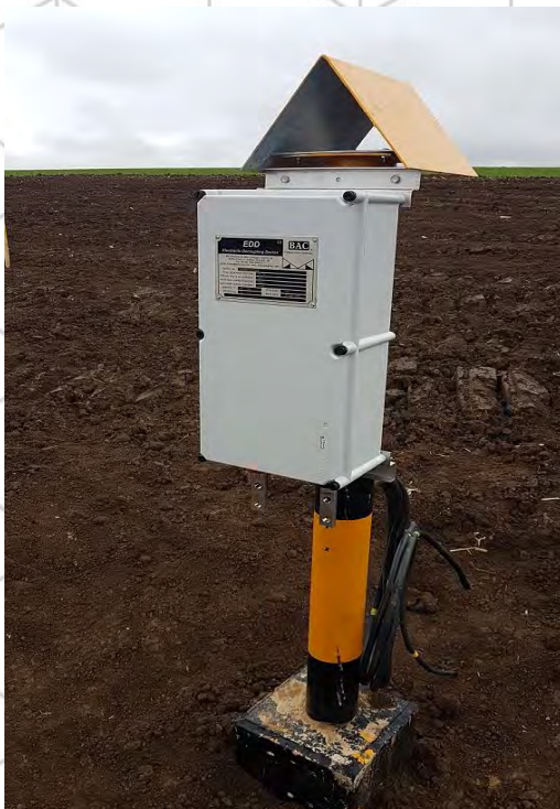
Solid State Surge Divertors for AC Mitigation
