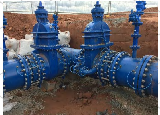
Pipeline continuity bonding using the Easybond Mk II Pin Brazing system
