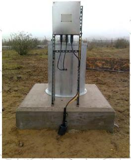
Typical Deep Well Anode Groundbed Installation
