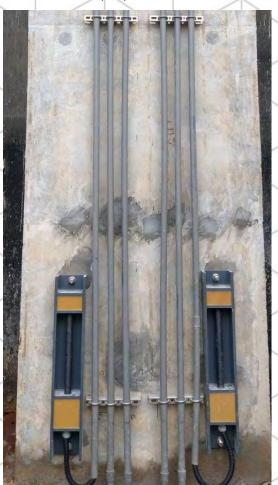
Mixed Metal Oxide Anodes for Water Intake Channel Structures
